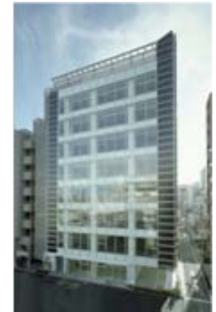
Shinjuku Tosei Building
