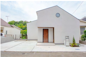
Example of ZEH construction
