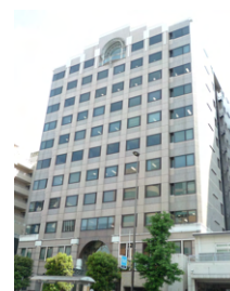
Narimasu Tosei Building
