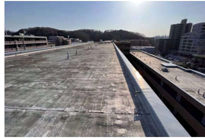
Rooftop where solar power generation equipment will be installed
