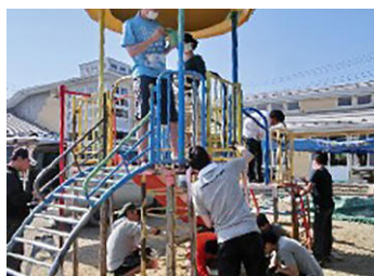
Rust removal and painting of nursery playground equipment
