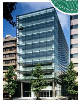
Toranomon Tosei Building
