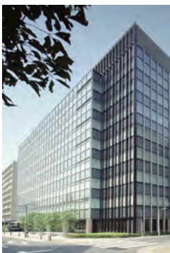
Kamata Tosei Building
