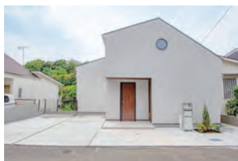
Example of ZEH construction
