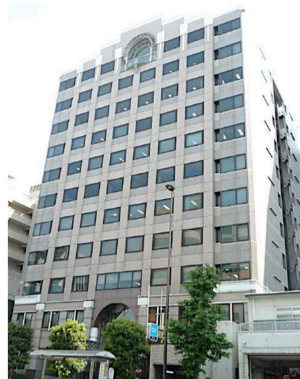
Narimasu Tosei Building
