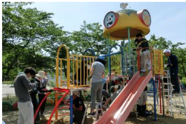
Rust removal and painting of nursery playground equipment
