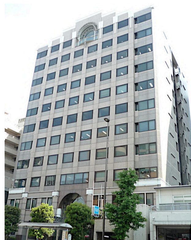
Narimasu Tosei Building
