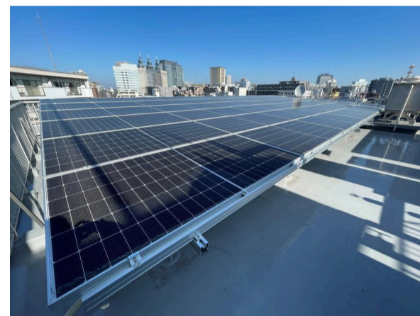
Solar panels installed on the rooftop
