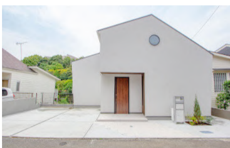
Example of ZEH construction
