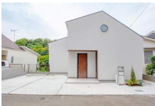
Example of ZEH construction
