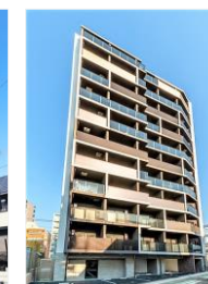
The Palms Yokohama-hiranumabashi (Rental apartment)
