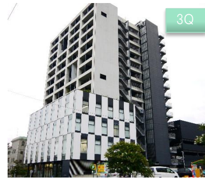
Chiba Minato Complex Facility (Commercial • Office • Residence)
